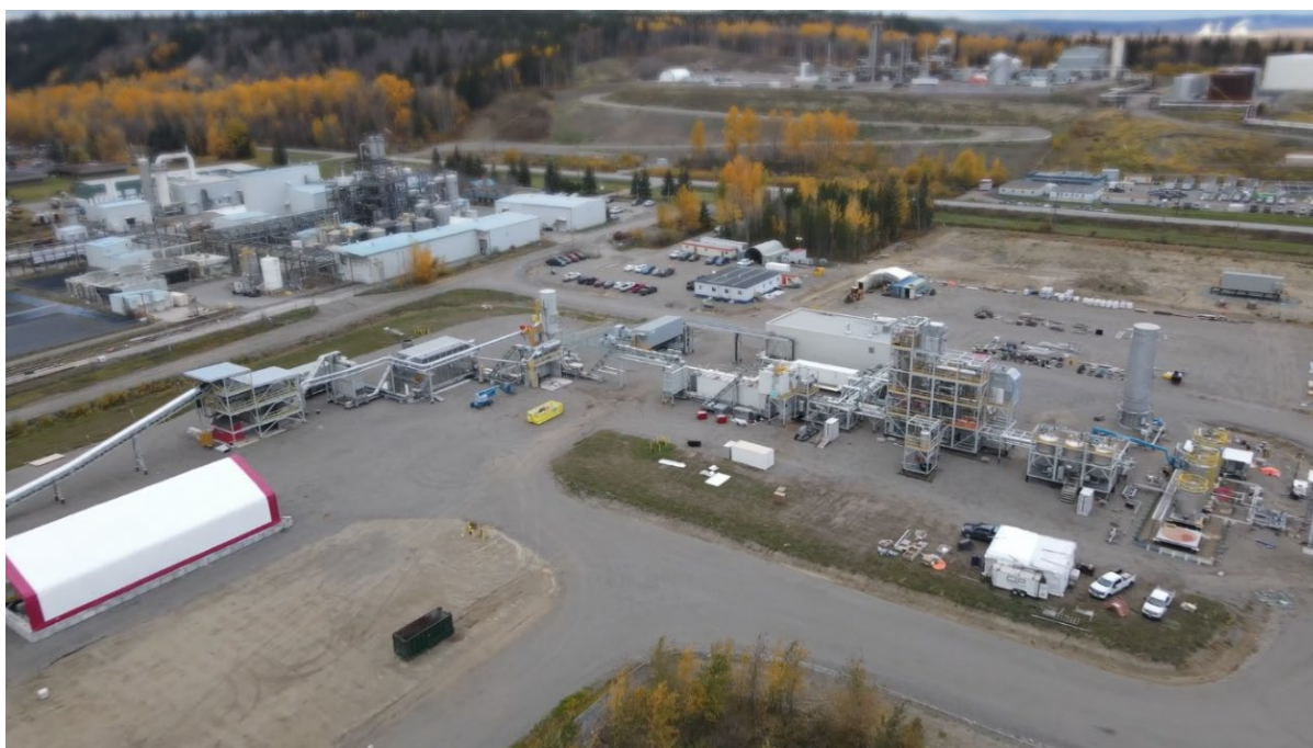
Figure 12: CS2 facility (front-end feedstock step on left and core Cat-HTR™ modules on the right)
